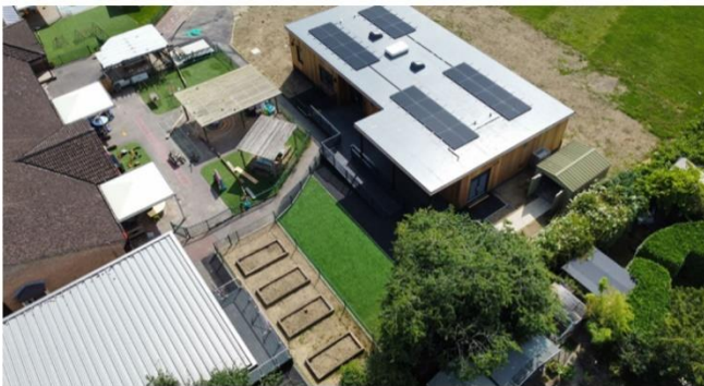
Image of the SEN Unit block and the new all-weather external play and gardening areas at St Matthews Church of England Primary School in Redhill.
