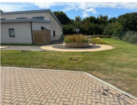
Image of the new 6th Form block at Woodfield School with external landscaping completed in Merstham
