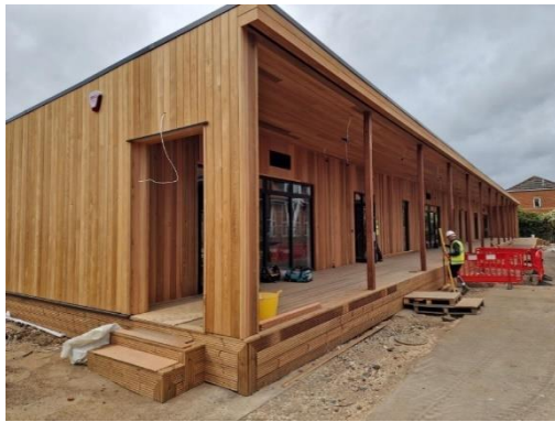
Image of the exterior of the new timber clad three classroom SEN Unit block at Stepgates Community School nearing completion in Chertsey.
